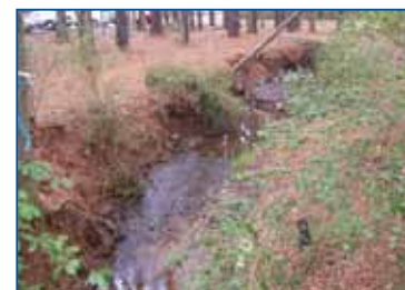
Typical streambank erosion and undercutting prior to restoration.
