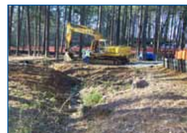
Project begins with site clearing and erosion and sediment control BMPs.
