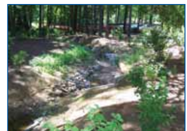
View of completed brush mattress and VRSS soil bio-engineering.
