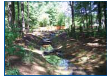
View of culvert crossing after removal with rock vanes in place.
