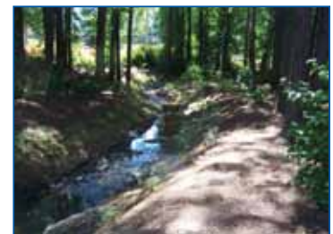
Riparian buffer vegetation installation completed.
