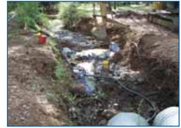
Installation of rock vane grade control.
